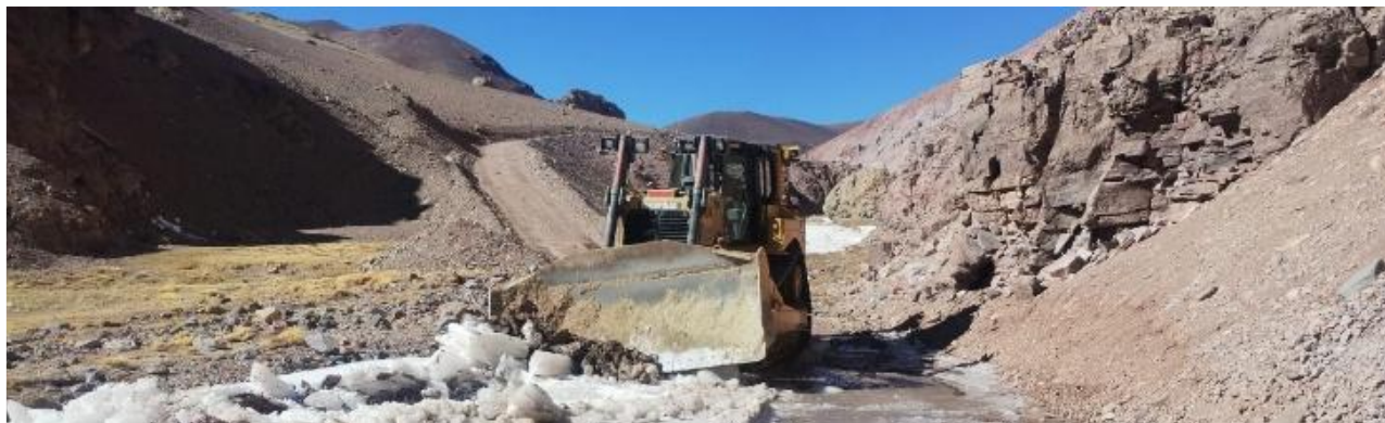
Figure 1 – Bulldozer clearing existing tracks of snow and rock debris en route to the TMT camp.
